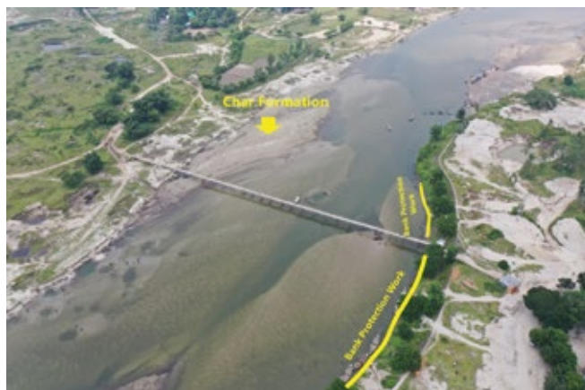
Bank Protection Work and Char Formation at Mirgarh Wooden Bridge, Panchagarh (Karatoya River)
