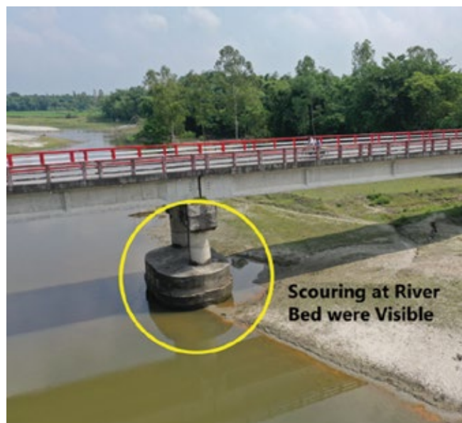
Overall Site Condition at Langolerhat Bridge (Ghagot River)
